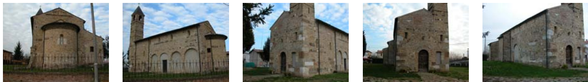
Figure 3: Some images (out of 22) of the Pozzoveggiani church. The church is 7 x 16 m large in the planar dimensions while the height is between 8 m (main roof) and 17 m (the tower).
